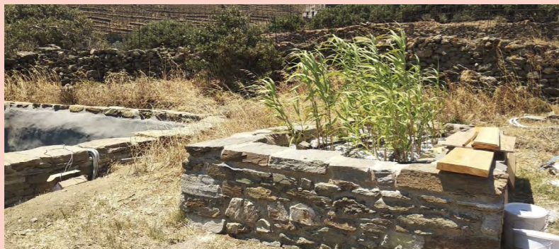
Constructed wetland operational
