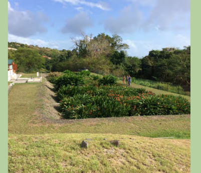
A treatment stage of constructed wetlands in Martinique (photo credit: INRAE)
