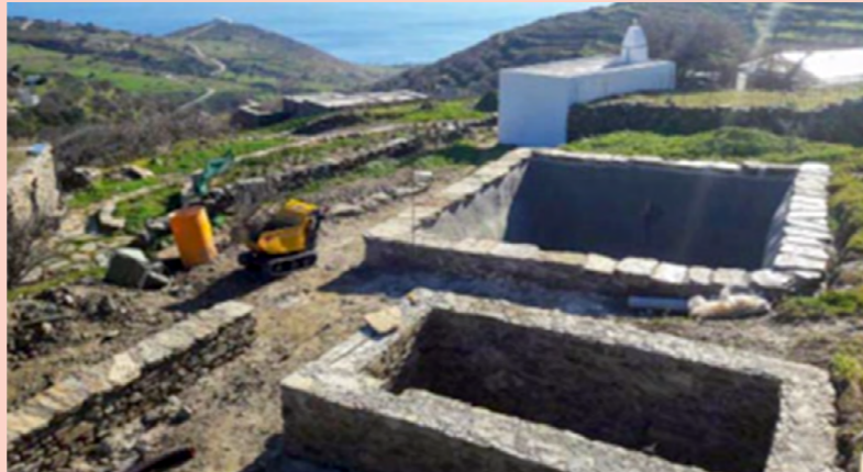
Constructed wetland and rainwater tanks under construction
